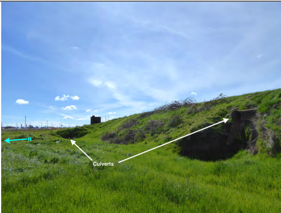
3. Water inputs to south end of parcel "detention basin"
